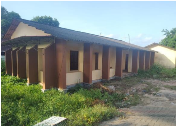
Figure 4: Site Picture_Side View
